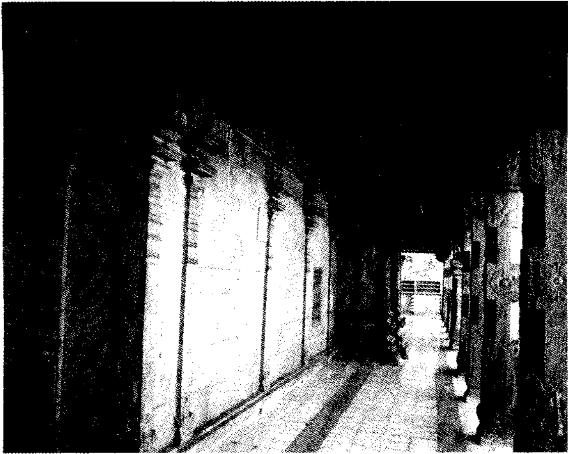
Fig. 93. Juma Masjid, Kilakarai - Rear Wall
