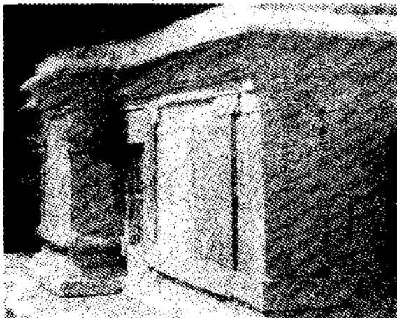
Fig. 21. External View of Mihrab
