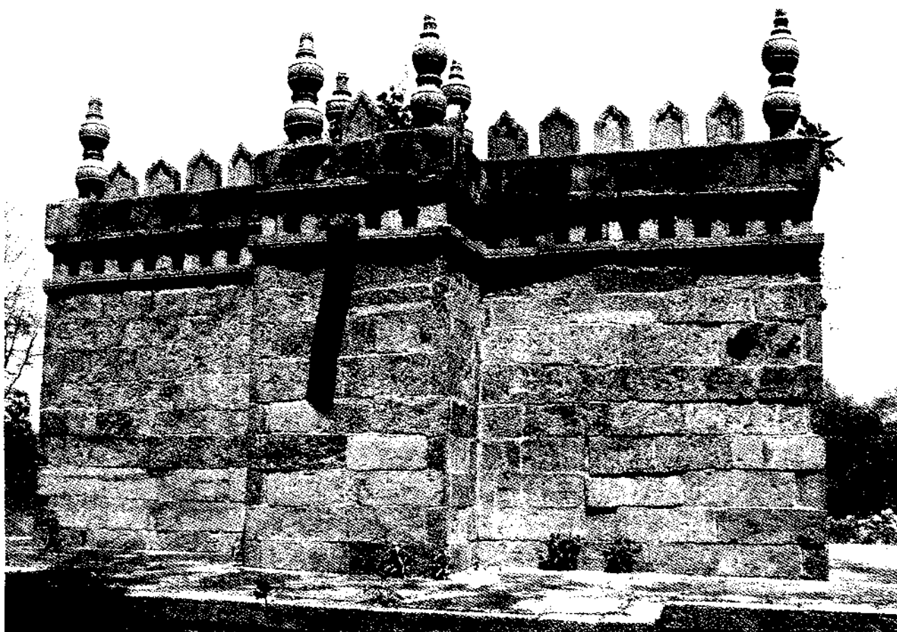
Fig. 64. Kallupalli - Valikantapuram - Rear View
