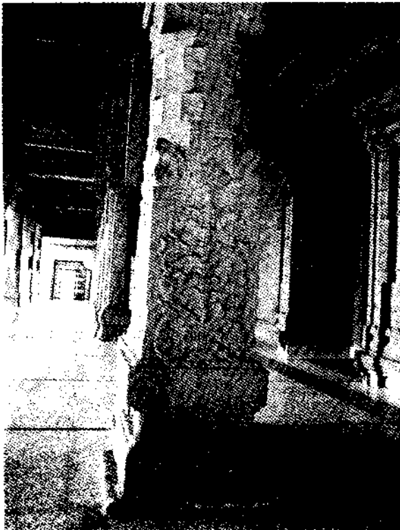
Fig. 83. Juma Masjid, Kilakarai - Pillar Base
